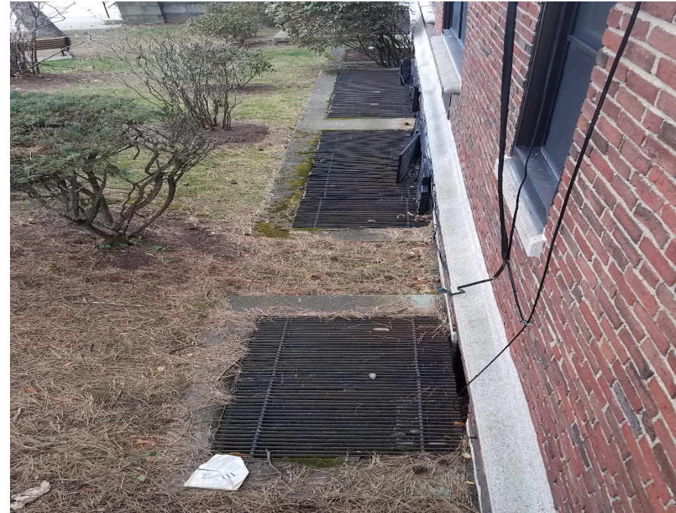
Figure 3: Window wells
